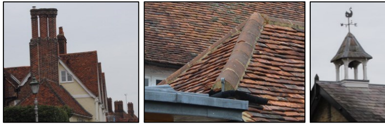
Figure 11 Examples of roof details in Much Hadham
